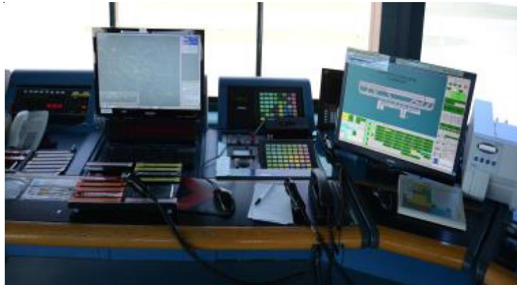
Fig 26. Bologna Airport TWR CWP
